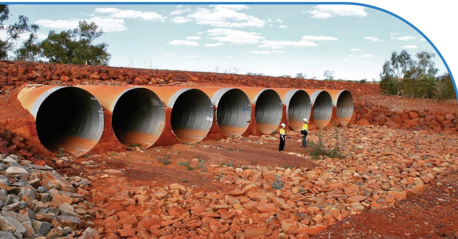
Image: CSP Culverts Installed for the access road.
