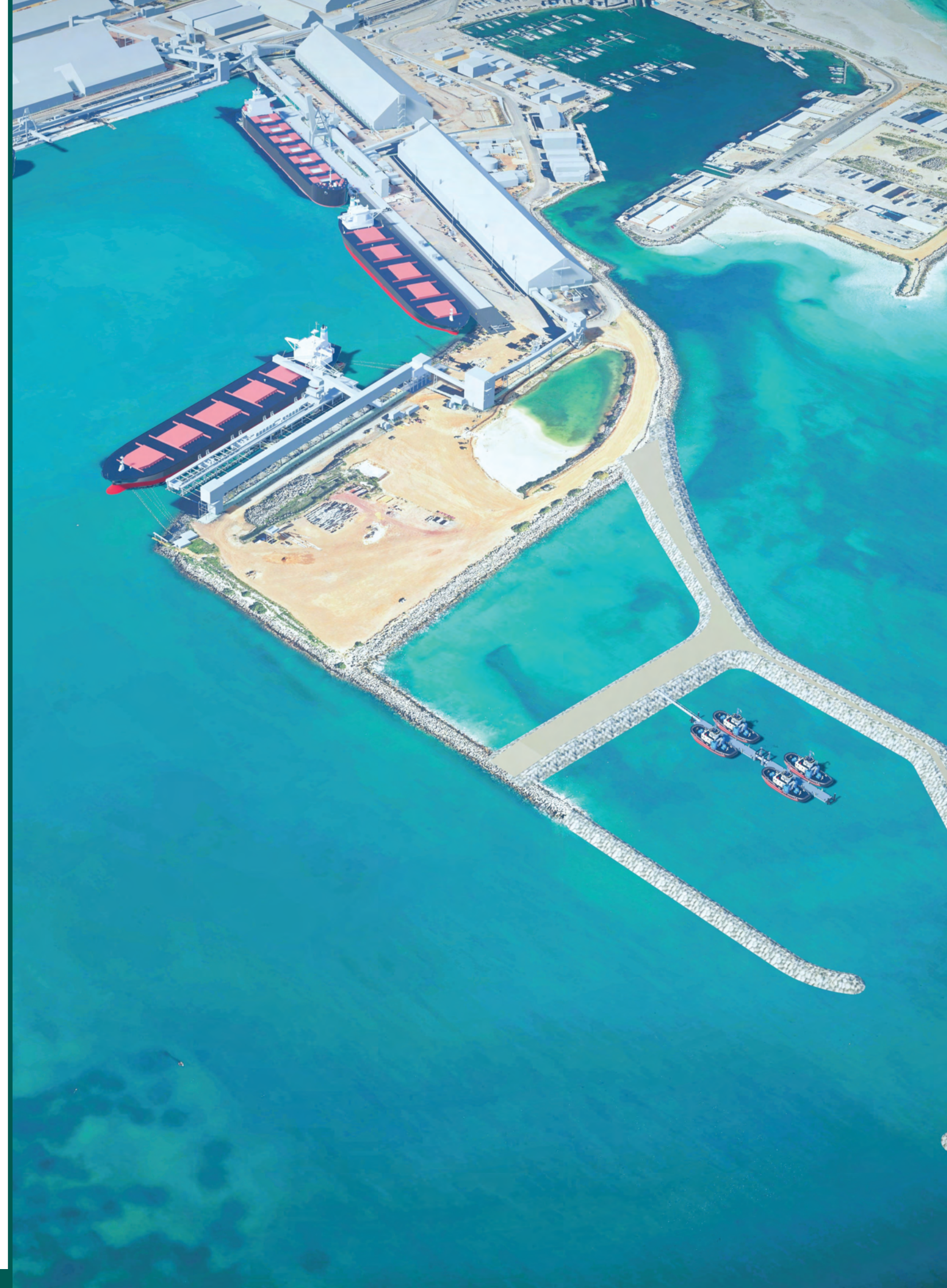
Image: Geraldton Port Maximisation Project (PMaxP), Western Australia.
