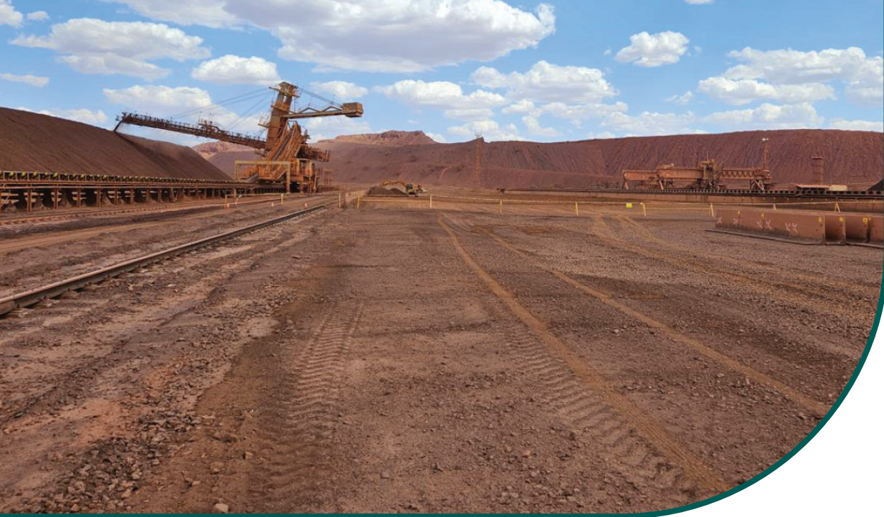
Image: Construction of the East Rockingham Waste to Energy facility, Rockingham WA.
