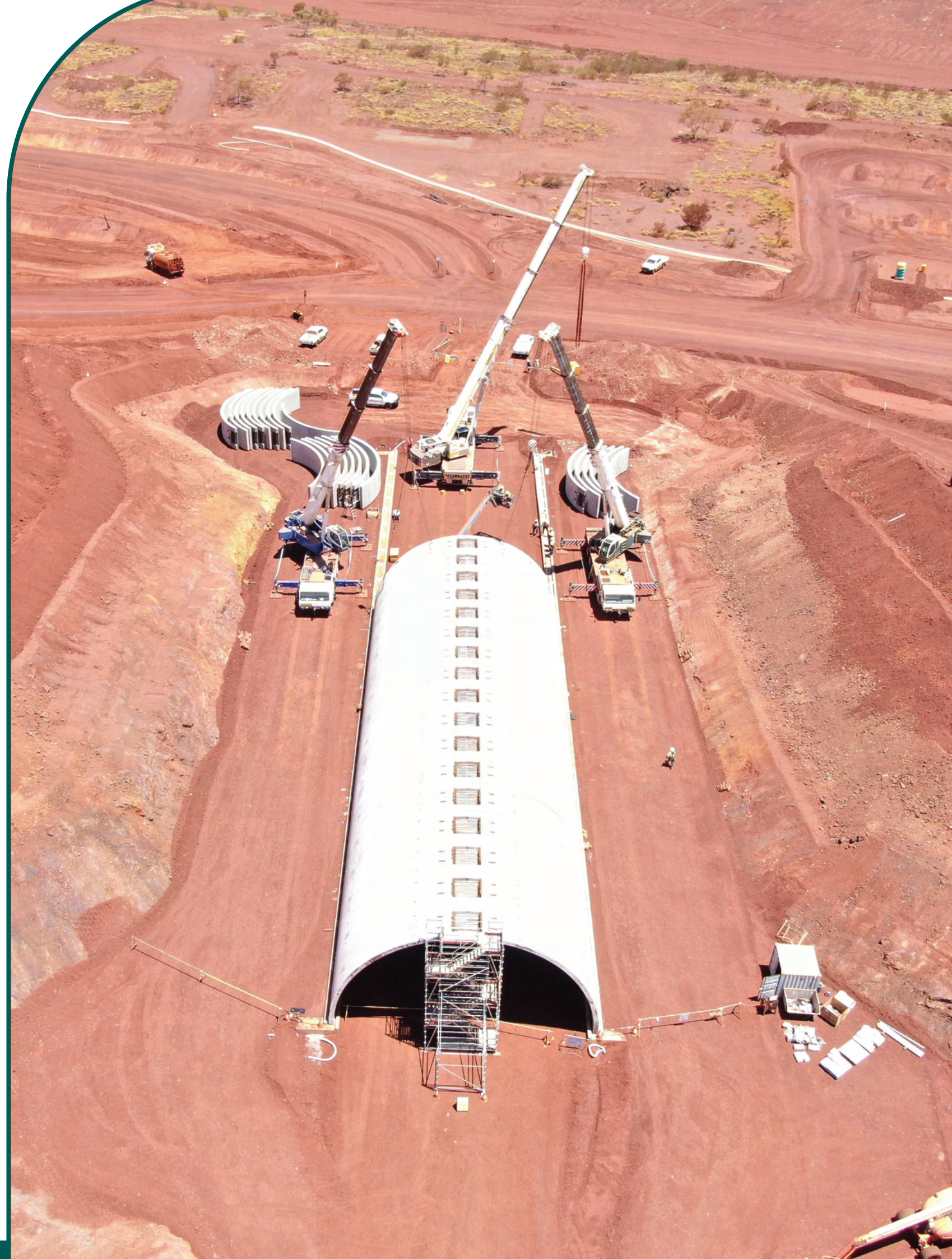
Image: White Quartz Road Construction, Pilbara WA.
