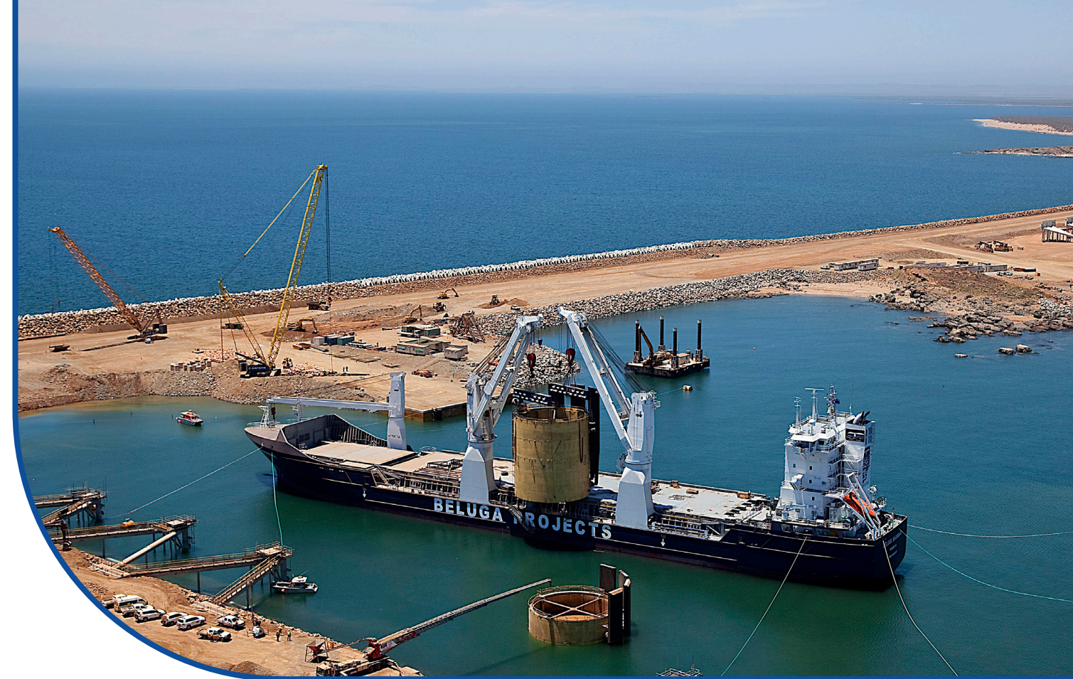
Image: Cape Preston Lift - Cape Preston, WA.
