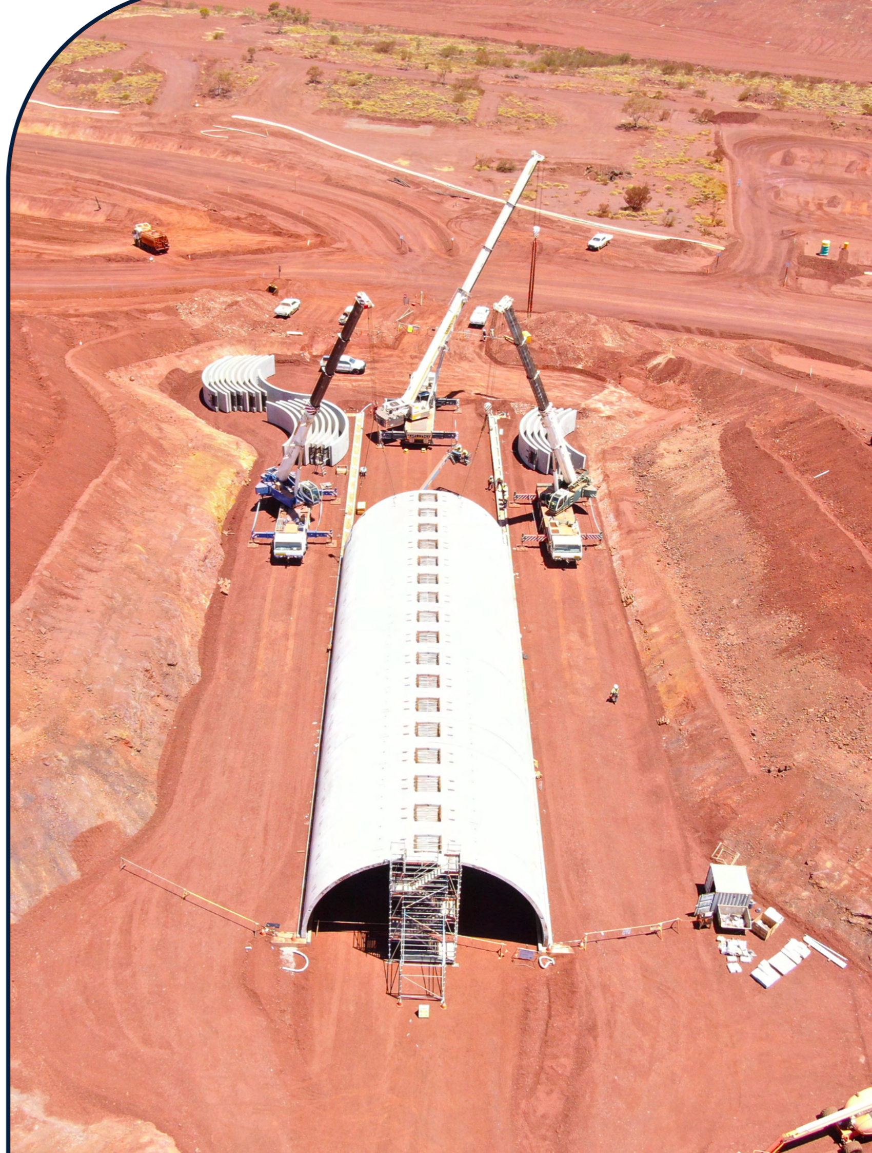
Image: White Quartz Road Construction, Pilbara WA.
