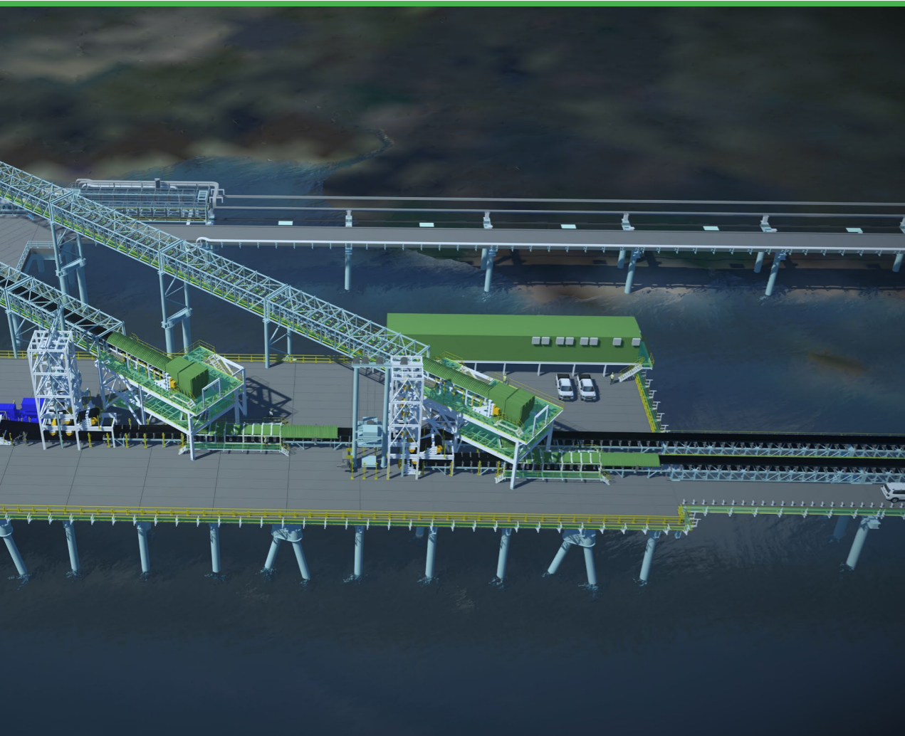
Image: Port Construction – Port Hedland, WA.
