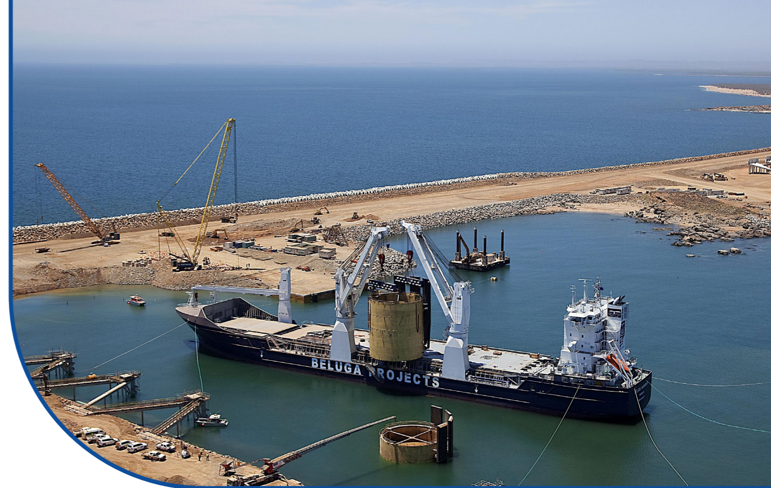
Image: Cape Preston Lift - Cape Preston, WA.
