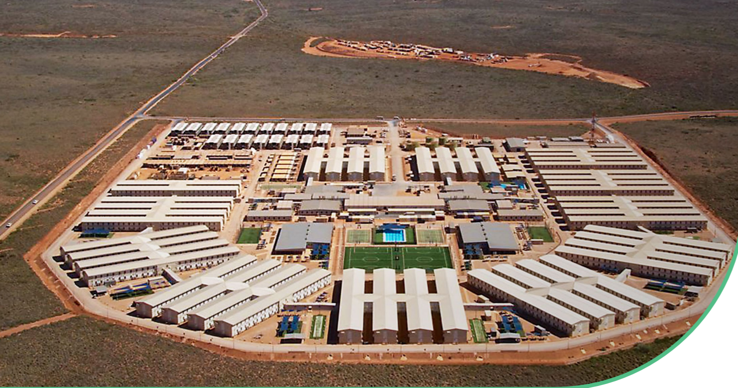
Image: Decmil Gorgon LNG Barrow Island Accommodation – Barrow Island, WA.
